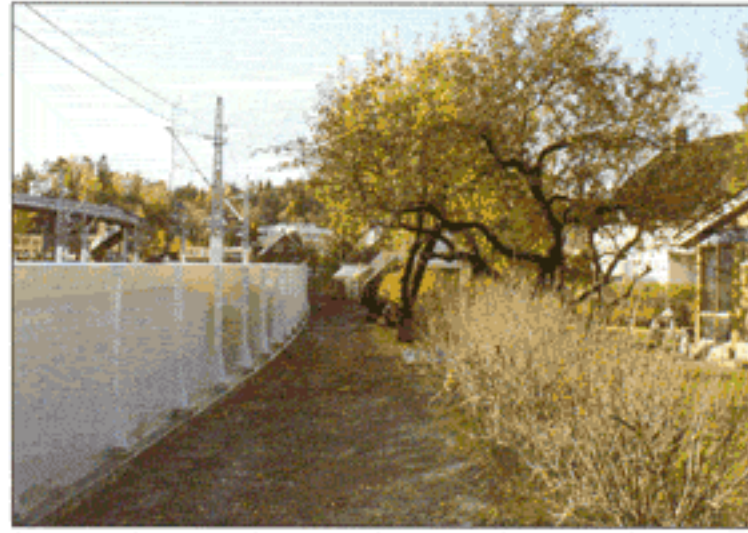
Noise barrier at railway. Oslo, Norway.
