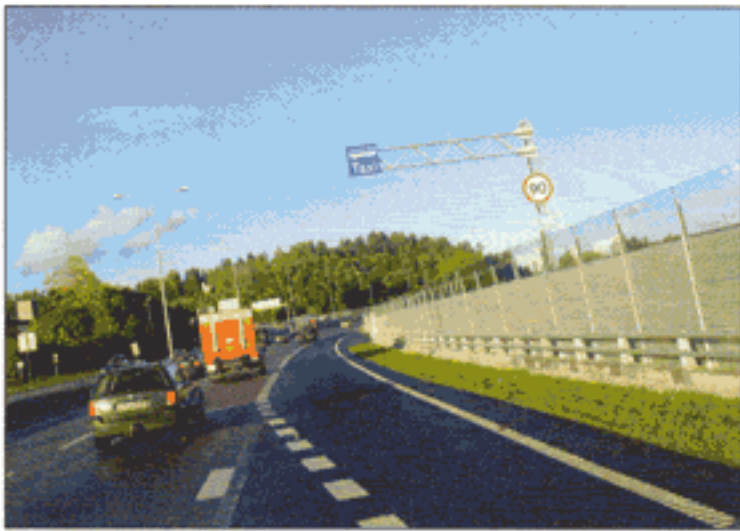
Noise barrier at road. Billingstad. Oslo, Norway.
