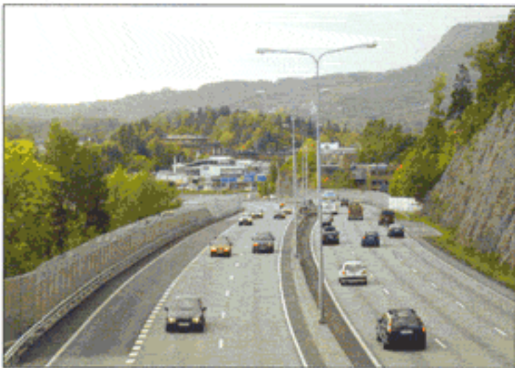
Noise barrier at road. Billingstad. Oslo, Norway.
