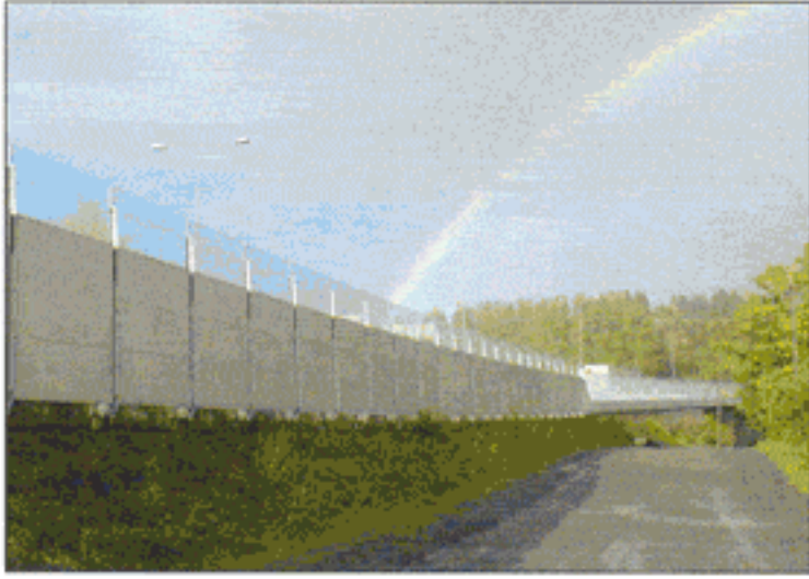
Noise barrier at road. Billingstad. Oslo, Norway.
