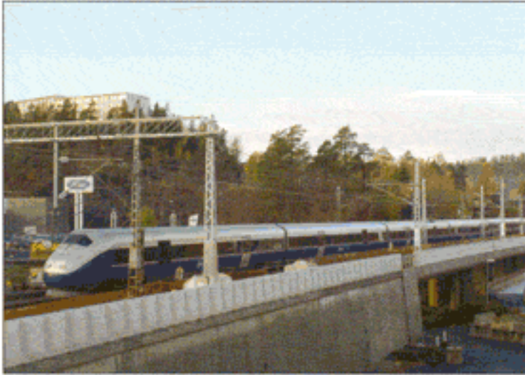
Noise barrier at railway. Oslo, Norway.
