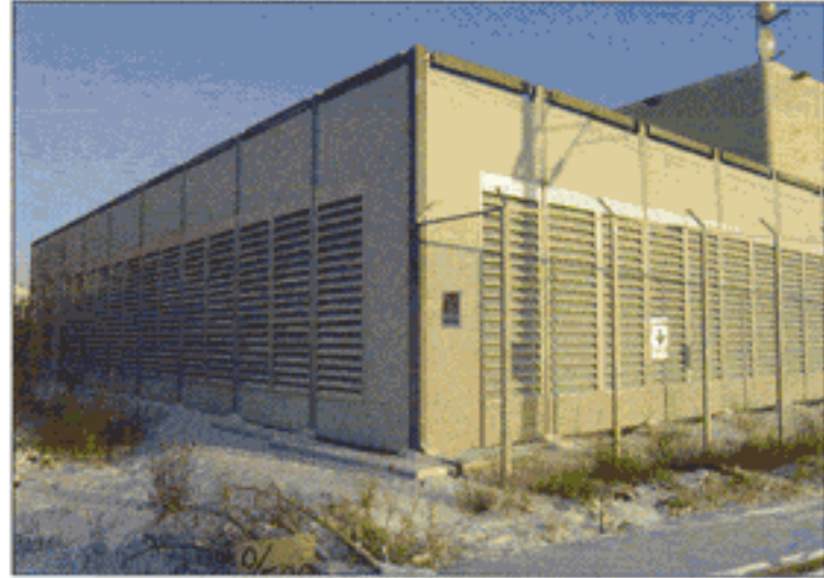
Noise barrier against radiator fan. Lunda Industrial area. Stockholm. Sweden.
