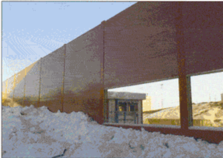
Noise barrier at steel plant. SSAB, Luleå, Sweden.
